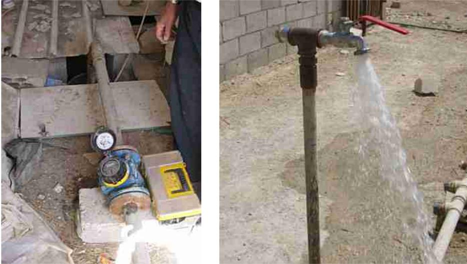
Figure A.3: Well head with flow meter and sampled tap of F3975
